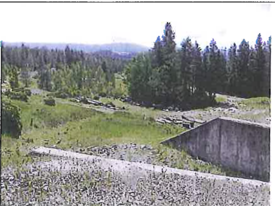
Looking south east from north end of dam across GEID property
